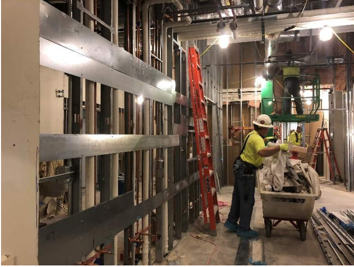
The new CS space having stud walls begin installed as well as the MEP roughs in / blocking. There is limited space within this area so all the crews must share one scissor lift or use ladders to reach high up work.
