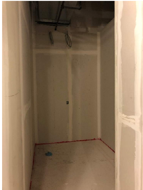
After all the in walls have been completed by the MEP trades as well as Findorff, the drywall installation proceeded and went by quickly! The crews can be seen taping the drywall in these photos preparing the wall for paint.
