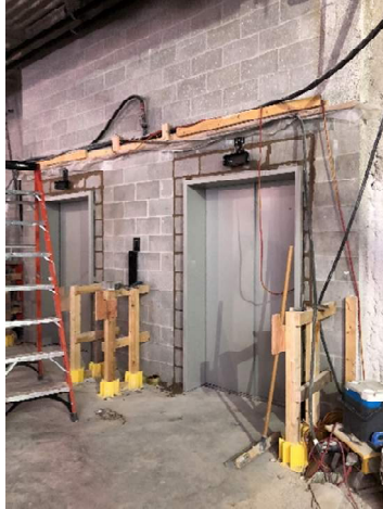
Findorff masons returned to the jobsite to installed the CMU block around the door frames of the elevators as seen in these photos.
