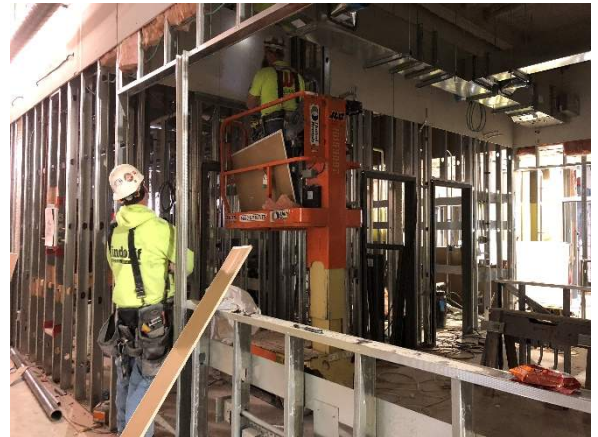
Drywall topping out installation occurring in the center core of the upper level Clinic / Med Surge addition.
