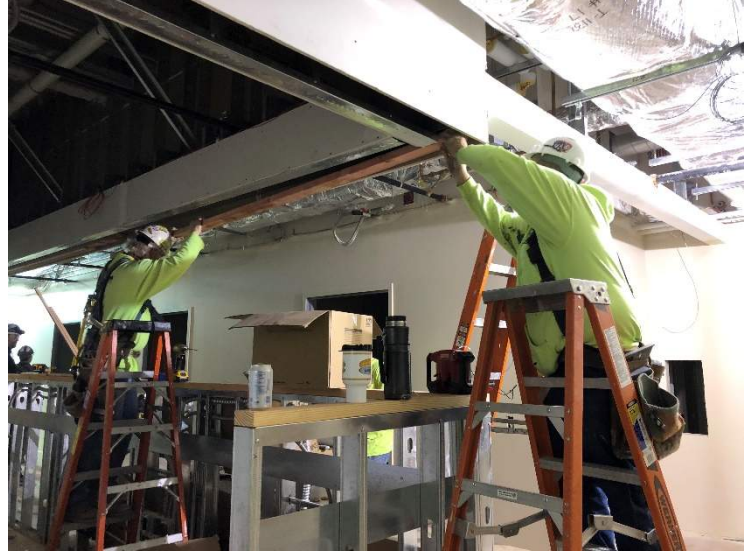
A view of a nurse station in the lower level Clinic / Med Surge addition. The Findorff carpenters are installed the blocking for the glass that will be installed here.
