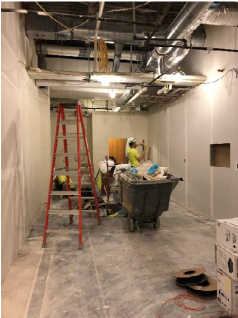
After all the in walls have been completed by the MEP trades as well as Findorff, the drywall installation proceeded and went by quickly! The crews can be seen taping the drywall in these photos preparing the wall for paint.
