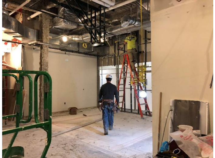
The new CS space having stud walls begin installed as well as the MEP roughs in / blocking. There is limited space within this area so all the crews must share one scissor lift or use ladders to reach high up work.
