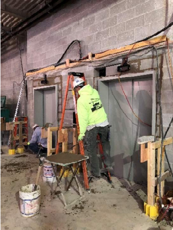
Findorff masons returned to the jobsite to installed the CMU block around the door frames of the elevators as seen in these photos.
