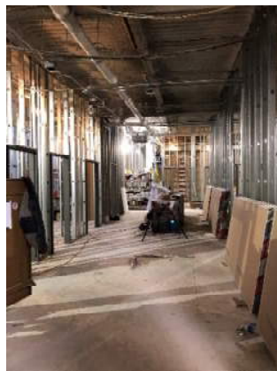
Various views of the framing and MEP rough ins down the long corridors of the lower level Clinic / Med Surge addition
