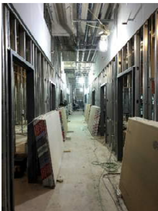
Various views of the framing and MEP rough ins down the long corridors of the lower level Clinic / Med Surge addition
