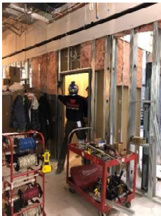
Various views of on going construction in the lower level Clinic / Med Surge addition. From left to right, photo 1: the first rooms to be drywalled are electrical closets so panels may be mounted and conduits piped, photo 2: MEP rough ins must be completed before drywall installation, photo 3: drywall is installed on one side of a wall then insulation in the middle of the walls, and photo 4: the corridor is ready for drywall!!
