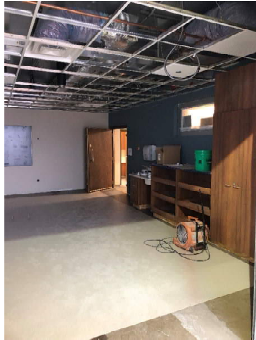
The MRI room is almost complete! The photo of the left depicts the process of laying the sheet vinyl floor down. First the vinyl is measured and cut appropriate then glue is laid on half the floor, then each sheet is pulled over the glue followed by pushing a heavy roller over the floor to ensure it properly adheres to the glue. The photo of the right is the final laid floor.
