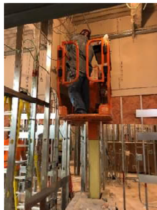
Various views of on going construction in the lower level Clinic / Med Surge addition. From left to right, photo 1: the first rooms to be drywalled are electrical closets so panels may be mounted and conduits piped, photo 2: MEP rough ins must be completed before drywall installation, photo 3: drywall is installed on one side of a wall then insulation in the middle of the walls, and photo 4: the corridor is ready for drywall!!
