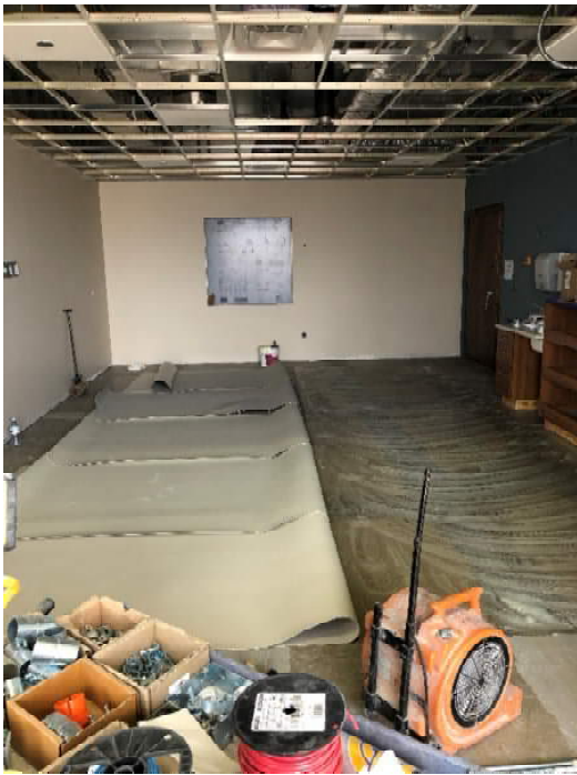
The MRI room is almost complete! The photo of the left depicts the process of laying the sheet vinyl floor down. First the vinyl is measured and cut appropriate then glue is laid on half the floor, then each sheet is pulled over the glue followed by pushing a heavy roller over the floor to ensure it properly adheres to the glue. The photo of the right is the final laid floor.
