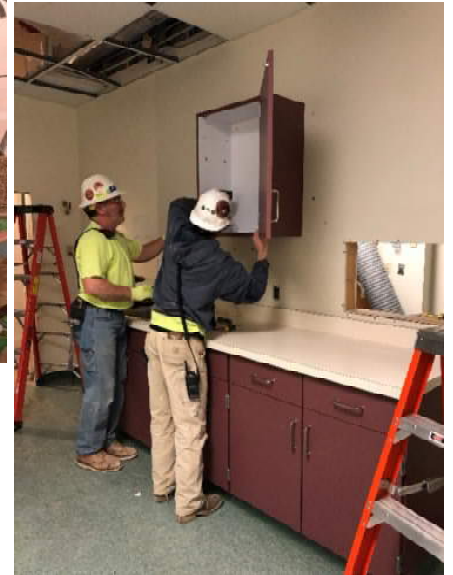
Light demolition within the old CS department.
