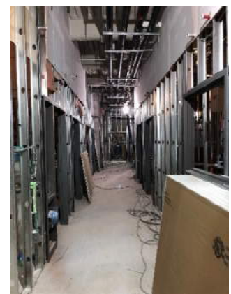
Various views of on going construction in the lower level Clinic / Med Surge addition. From left to right, photo 1: the first rooms to be drywalled are electrical closets so panels may be mounted and conduits piped, photo 2: MEP rough ins must be completed before drywall installation, photo 3: drywall is installed on one side of a wall then insulation in the middle of the walls, and photo 4: the corridor is ready for drywall!!
