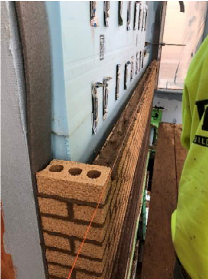
The skinny orange string seen on the exterior brick installation photo above, reaches across the entire façade and allows the masons to keep a level check at all times while installing the brick.
