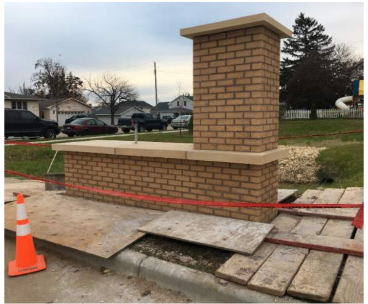
The base for the new monument sign at the North side of GRHC near Oak Street. Soon this sign base will also have the sign to go with it!
