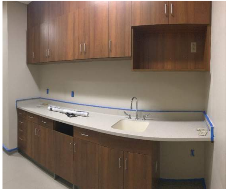
The nourish station that was installed in the Education Area. It will soon receive a few appliances, and the final accessories will be installed.
