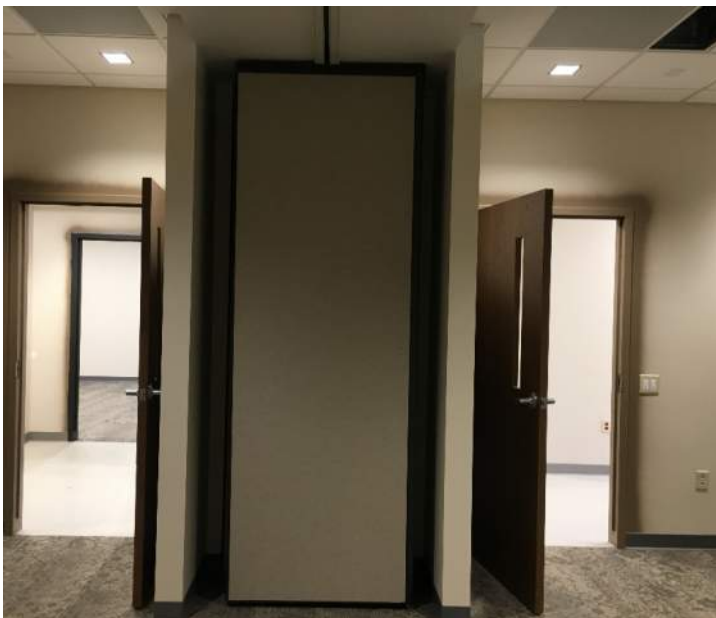
Folding partitions were installed in both of the classrooms down in the Education area. These will help separate the rooms to allow for multiple groups to work at one time.
