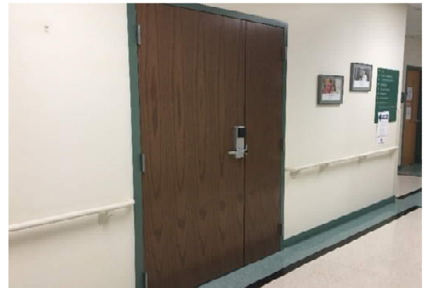
Doors for the new IDF 7 room have been added and the finishes in the area touched up.
