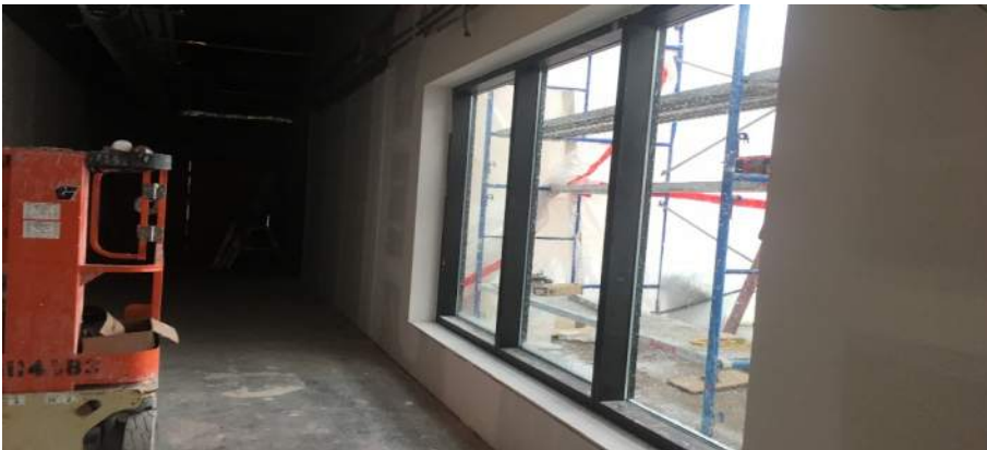
New windows and doors are added in the hallway that leads from the Ambulance Garage to the new Emergency Department.
