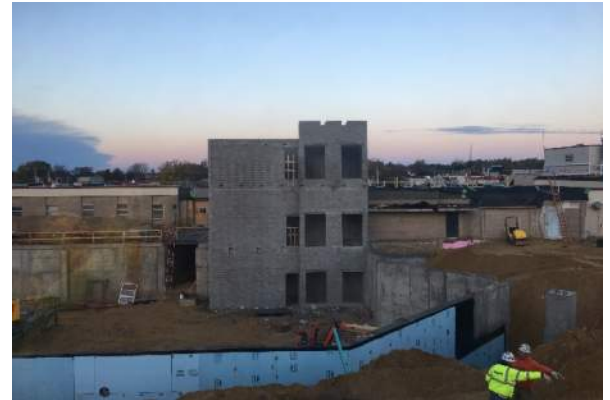
The elevator and stair shaft have been completed and will soon have usable stairs and an elevator inside!
