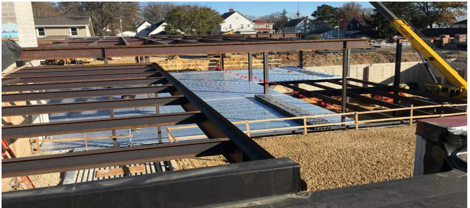
A view from the roof of the steel and deck being installed for the new Clinic / Med Surge addition. Here you can also see the courtyard area that will be accessible from inside of the building . This is located where the gravel is shown in the bottom right corner.
