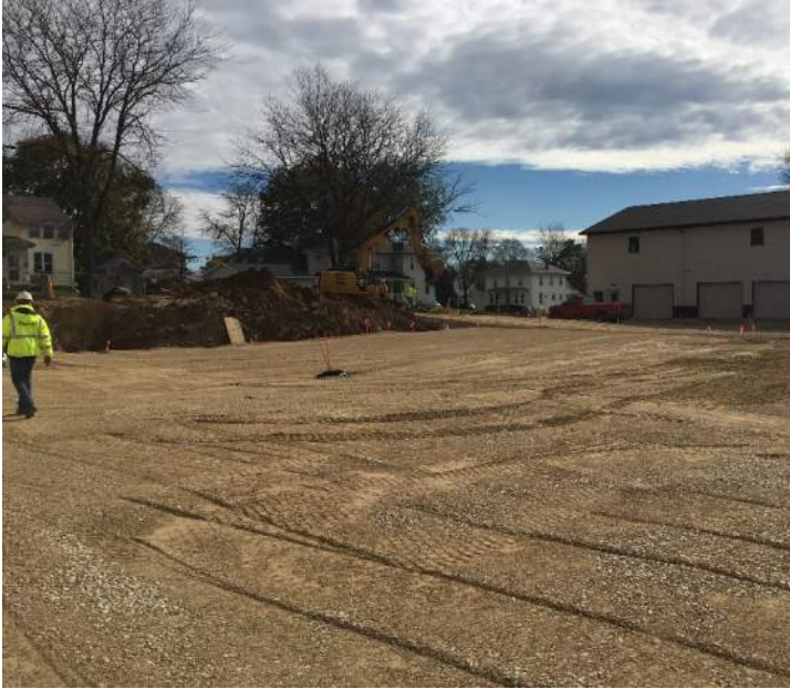
Grading for the new Rehab lot is underway. The final layout and materials for grading were installed last week.
