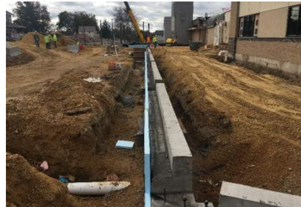
Footings, foundation walls, and underground plumbing is being installed for the new Main Street addition.
