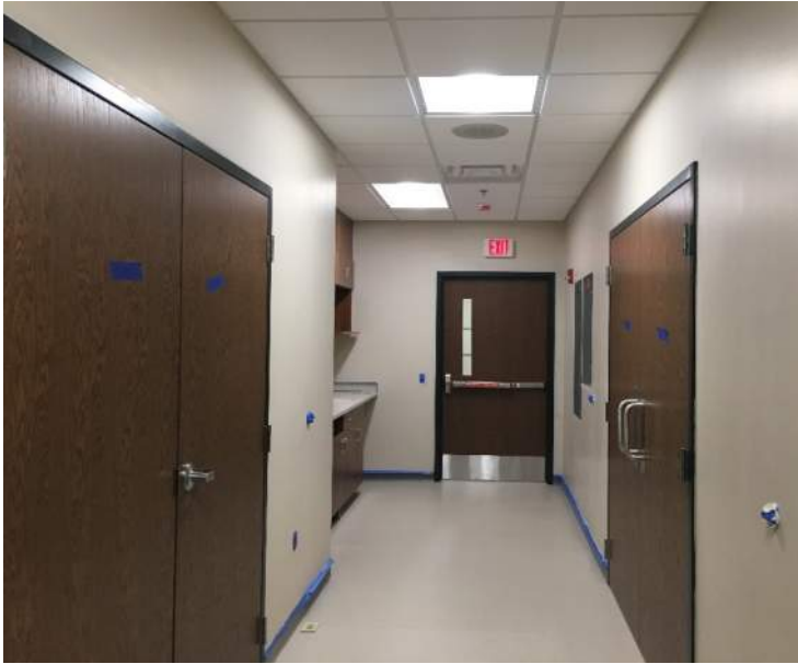
A view down the hall of the Education area that will open up to the existing facility in the lower level Clinic area.
